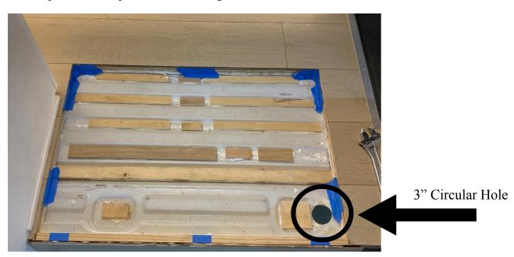
**Step 8:** Reinstall drain fixture onto shower pan ensuring tightness and good seal.
