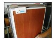
**Step 4: Slide new panel into frame, replace bottom retainer, and replace screws.**
