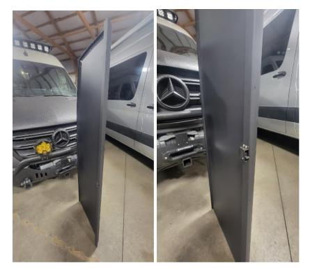
First, you will attach the rear panel to the right and left panels. The rear panel will be inside the side panels with the 5/8" support tabs on the outside of the shower. Stand up the left panel and back panel. Rest the rear panel against the inside of 5/8" tab of left panel. Tape can be used to hold pieces together until you get a rivet placed. Use provided rivets in 10 pre lasered holes to attach the left and rear panels together.
